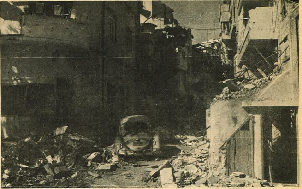
These ruins in Bourj Hamoud are typical of the type of destruction and desolation that have become common.
